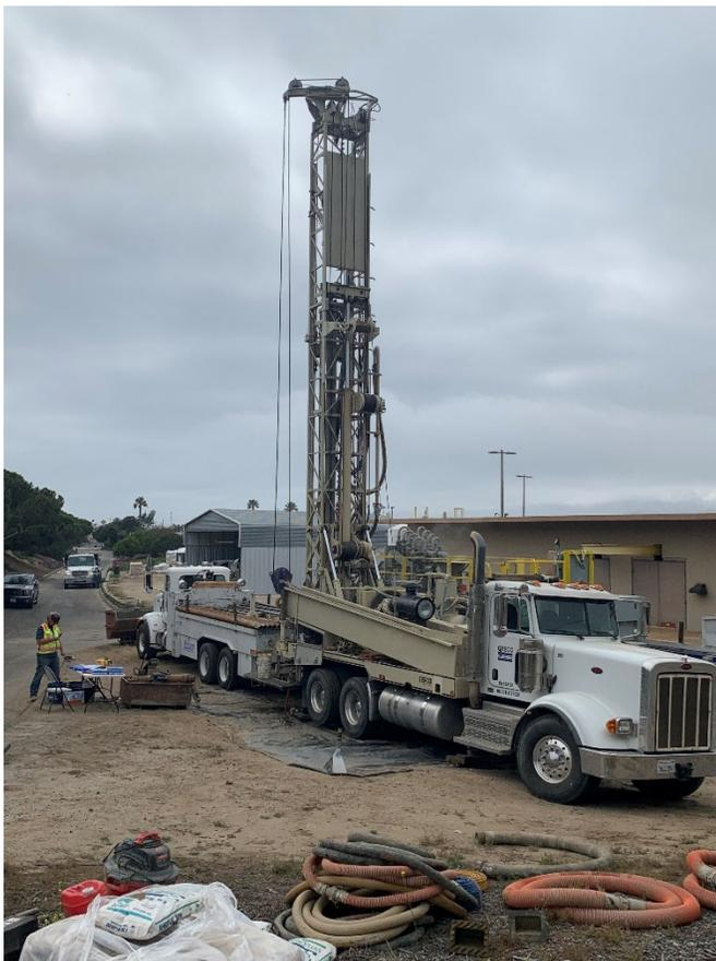
Photo 3. Mud rotary drilling setup. Pilot hole drilling in progress. Note geologist logging table on left.
