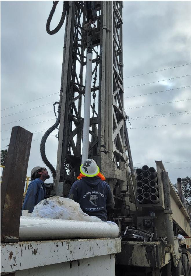
Photo 9. Installing PVC well casing.
