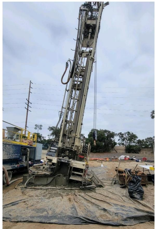
Photo 4. Drill rig leaning due to sinkhole formed during drilling activities.
