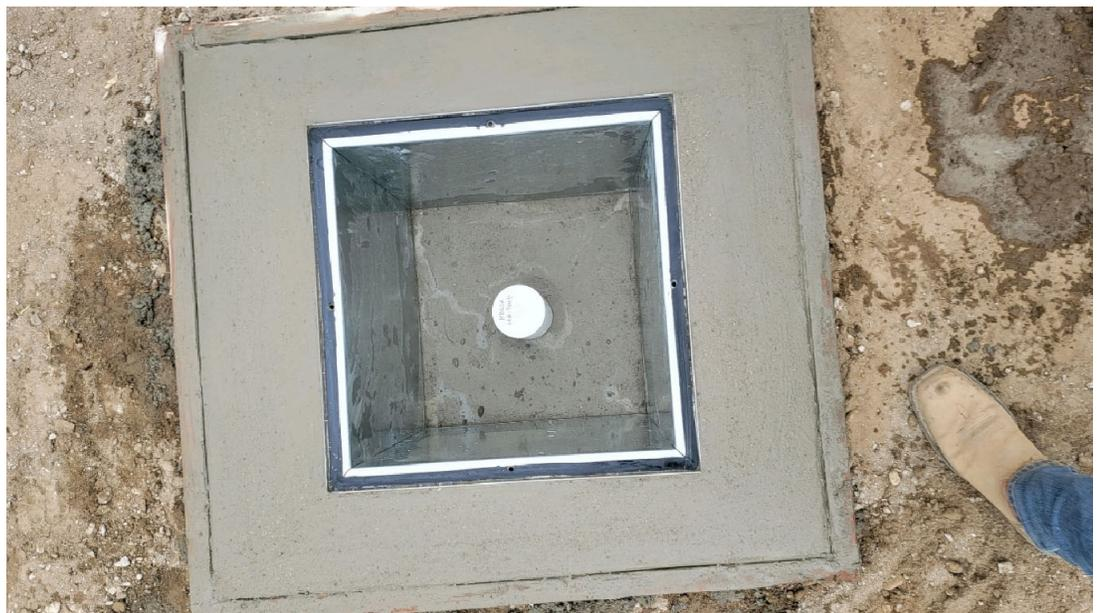
Photo 13. 2'x2'x2' traffic rated vault set in concrete (vault lid not in view).
