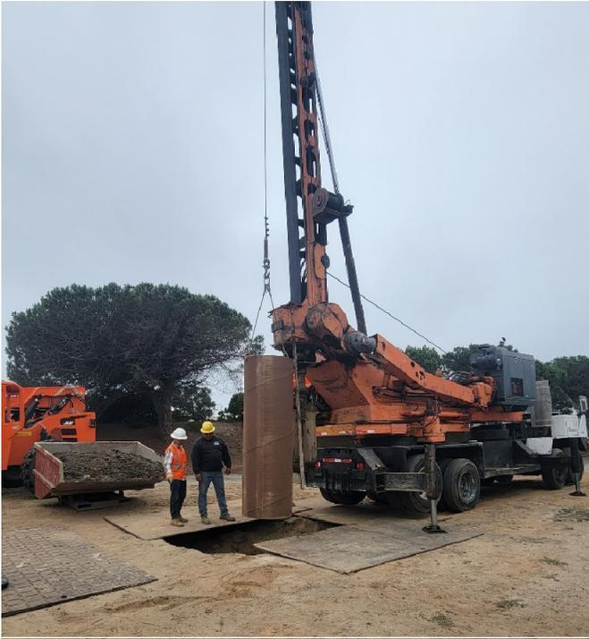
Photo 1. Installation of conductor casing
