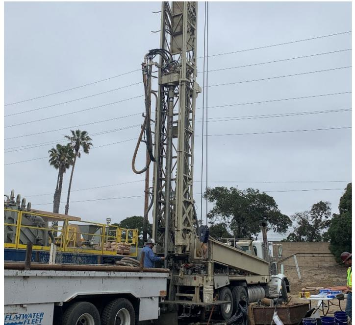
Photo 2. Mud rotary drilling setup. Pilot hole drilling in progress.
