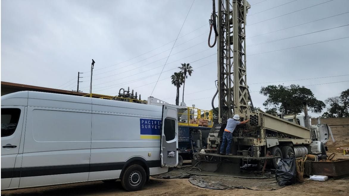
Photo 8. Performing geophysical survey of borehole to inform well design.
