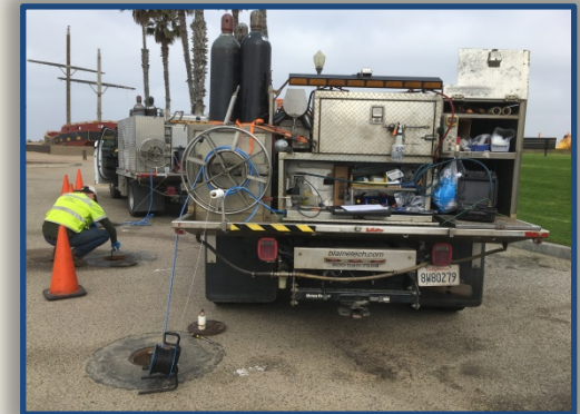
Groundwater sample collection from the Marina Park monitoring well
